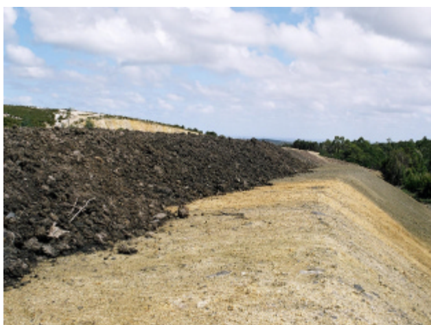
Plate 13: Organic matter on CWRD prior being spread.
