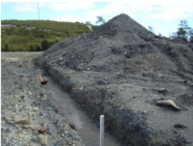
Plate 1: Stockpile surface drain.
