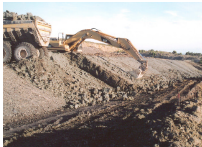
Plate 12: Application of clay on CWRD.
