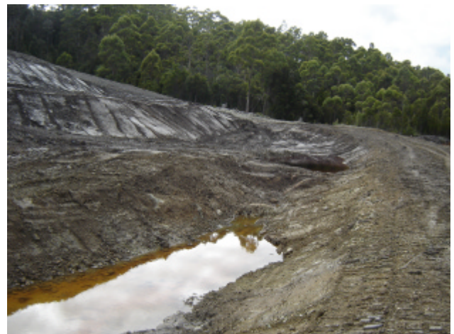
Plate 2: Silt traps at the base of STWRD.
