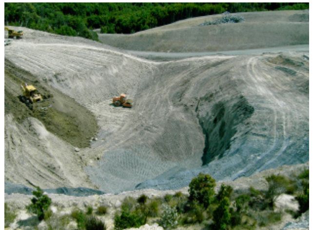
Plate 16: Compaction of waste material
